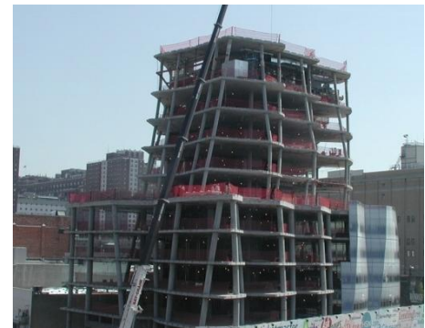
Figure 3: Flat-plate system during construction of the IAC Headquarters
